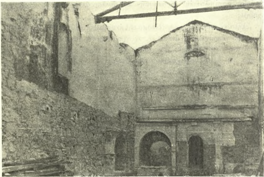
Εἰκ. 1. Ἀποψὶς τοῦ ἐσωτερικοῦ τοῦ ναοῦ ἀπὸ Α μετὰ τὴν μερικὴν ἀφαίρεσιν τῶν κονιαμάτων.
