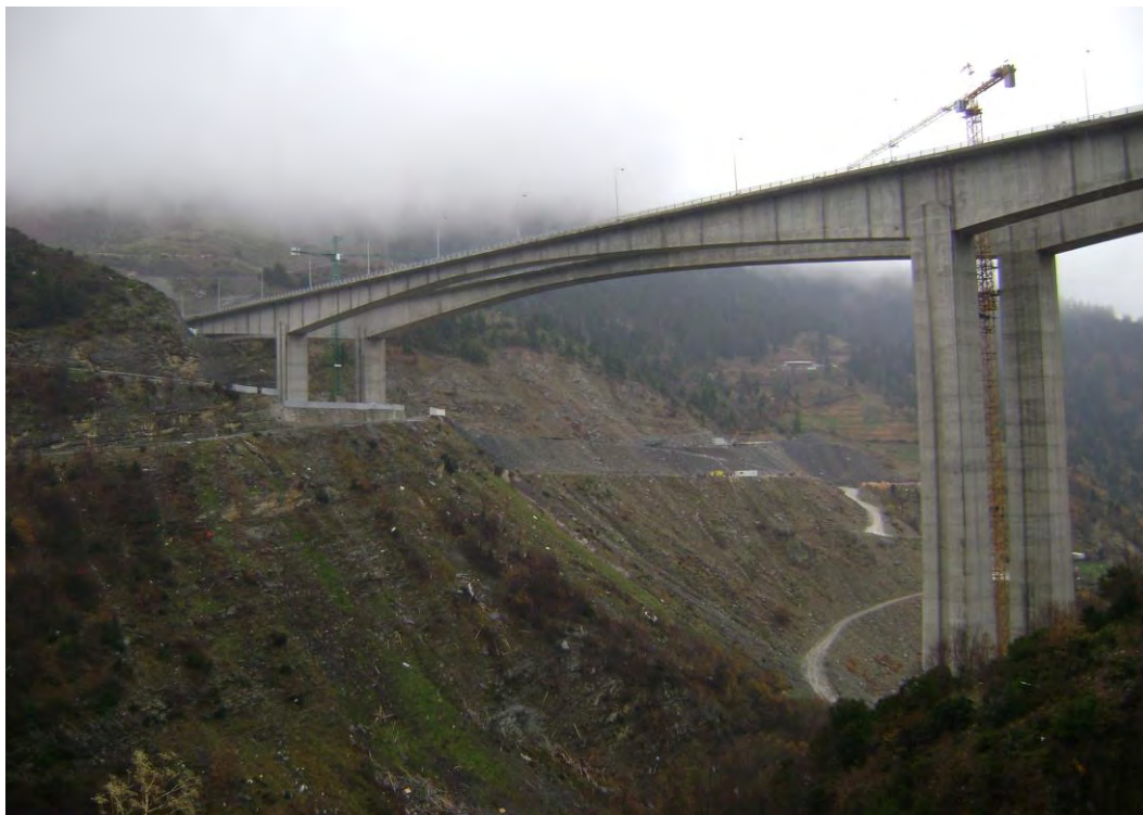
Figure 3.1: General View of Metsovo bridge.
