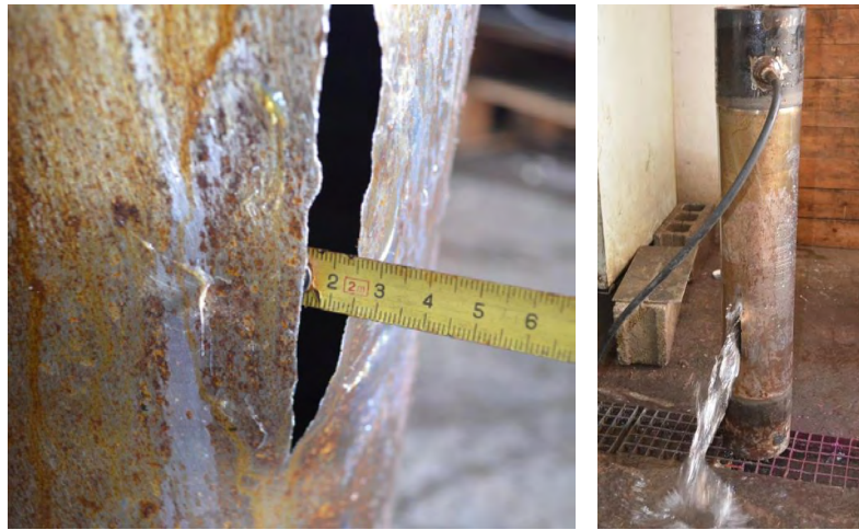
Figure 3-62: Rupture of perfect \text{Ø}165/3 pipe specimens; (a) thickness wall reduction at the critical region and (b) the location of the rupture.
