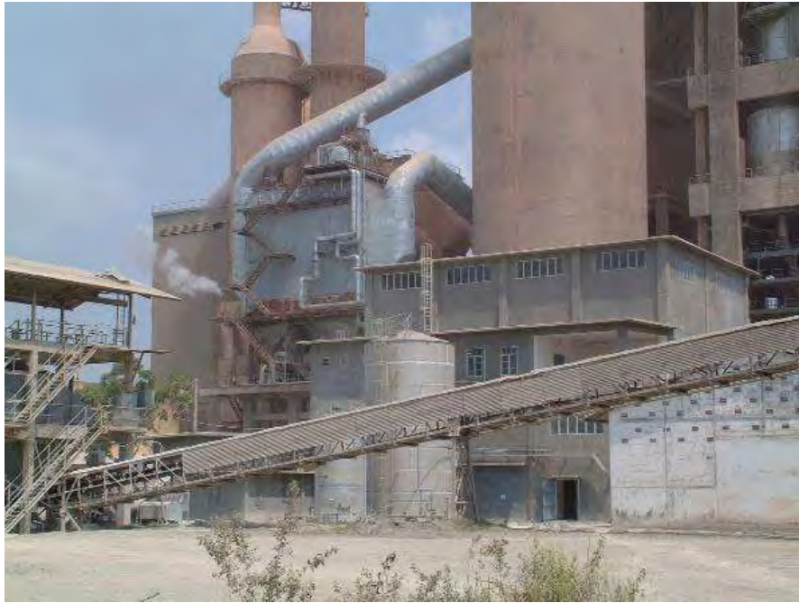
Figure 3.3: Preheater boiler & turbine / generator house installed by Kawasaki at Ha Tien plant in Vietnam
