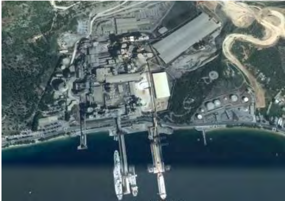
Figure 2.2: Volos cement plant
