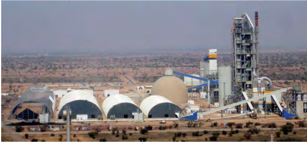
Figure 1.3: Italcementi's Ait Baha plant in Morocco
