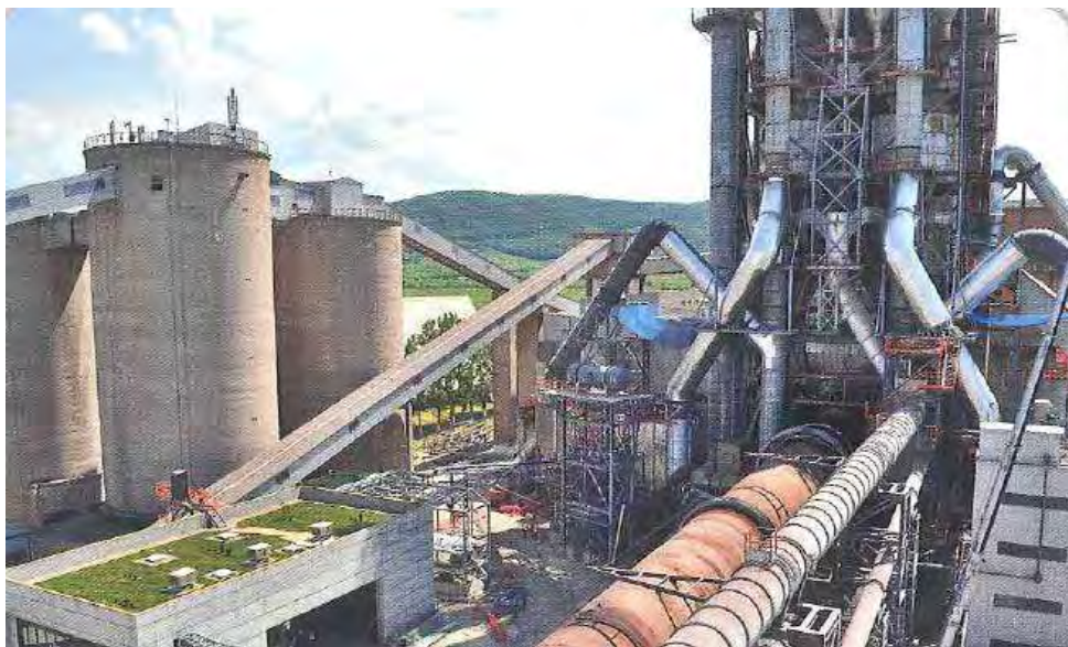
Figure 1.5: Holcim Alesd cement plant – Romania
