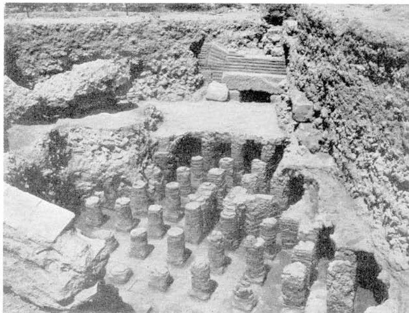
Corinth. Roman Bath: a. Part of west wall of Central Court, from east, b. Caldarium and hypocaust, from east
