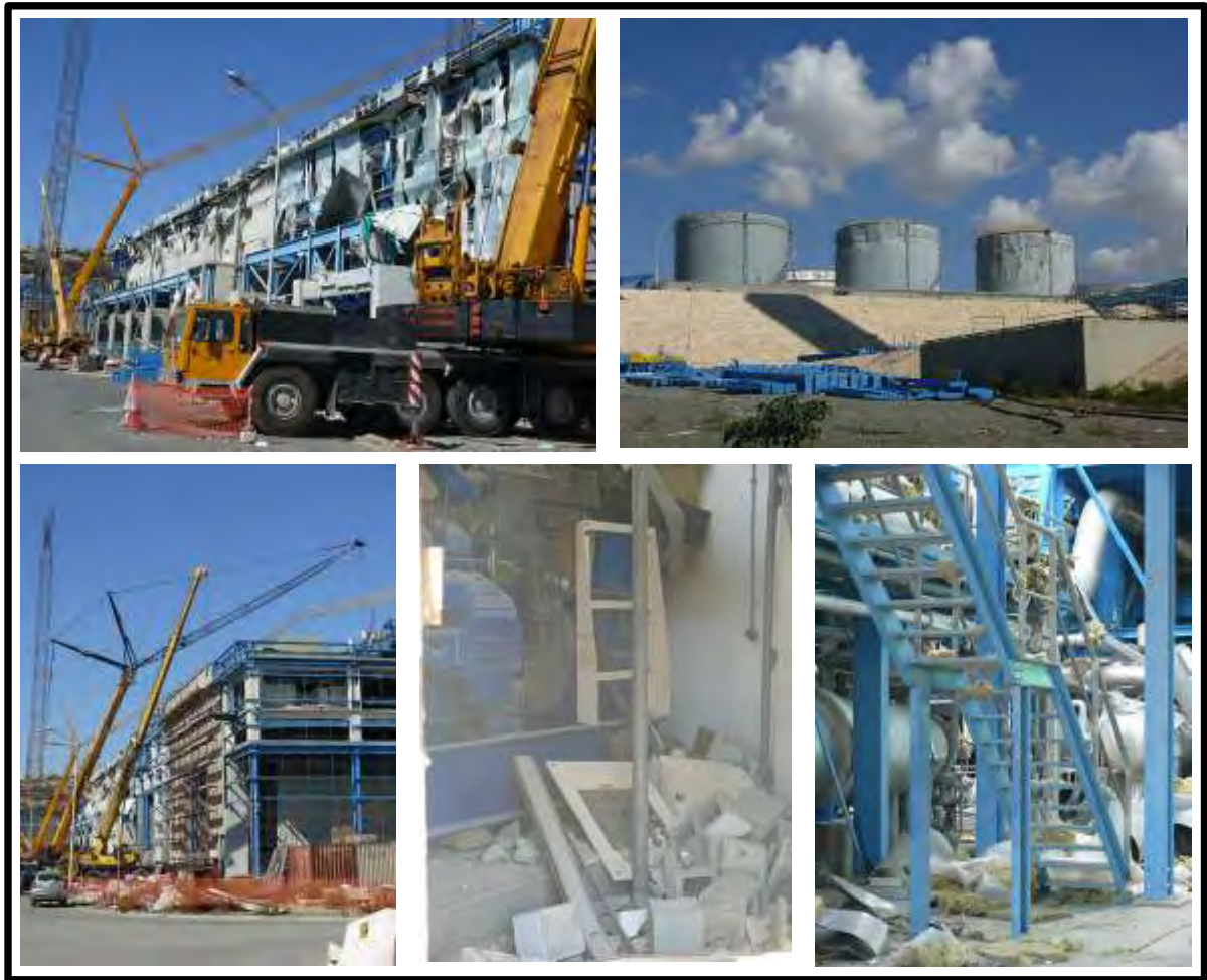
Figure 1. Pictures from Vasilikos Power Station (October 13th, 2011).
