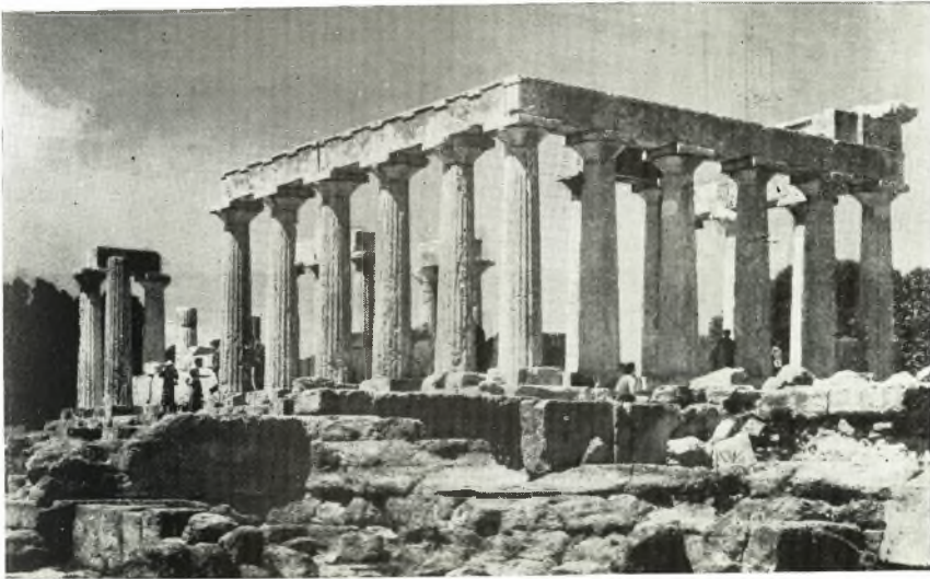
α. 'Ο ἐν Αἰγίνῃ ναὸς τῆς Ἀφαίας πρὸ τῶν ἐργασιῶν ἀναστήλωσεως τοῦ 1959.
