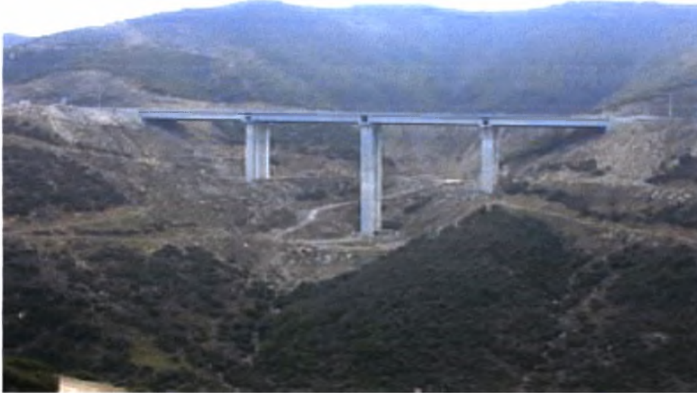
Figure 5.25: View of 2 nd Kavala bridge
