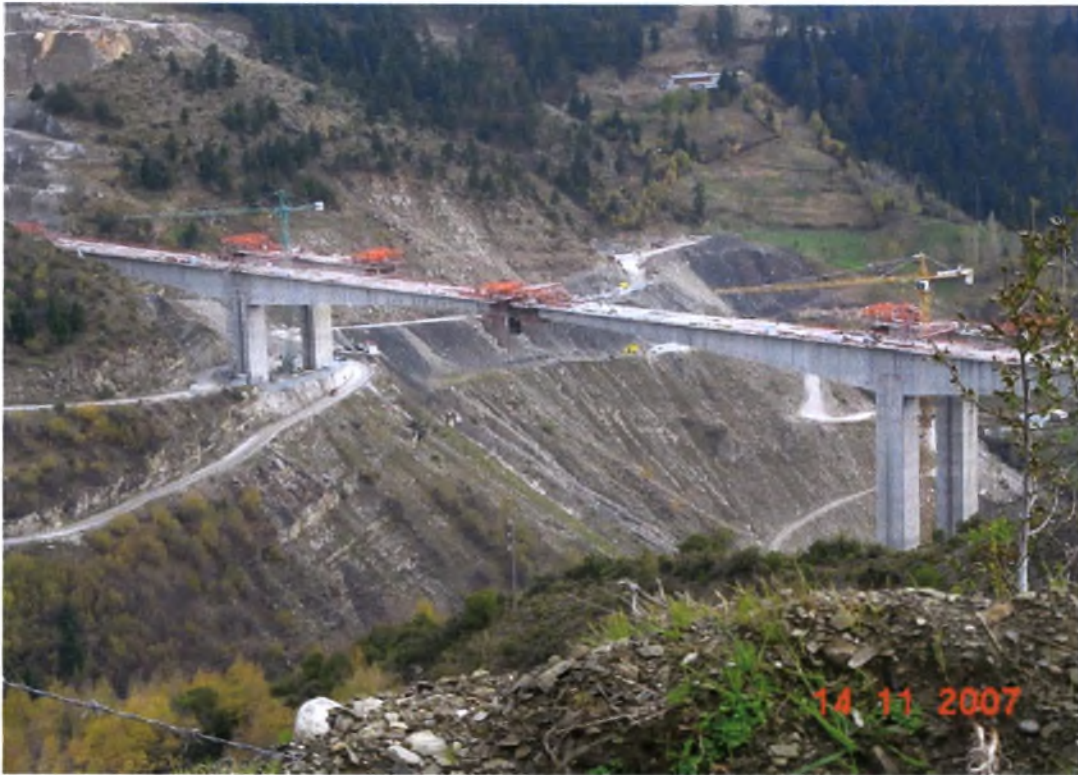
Figure 5.18: General view of under construction Metsovo ravine bridge (November 2007)
