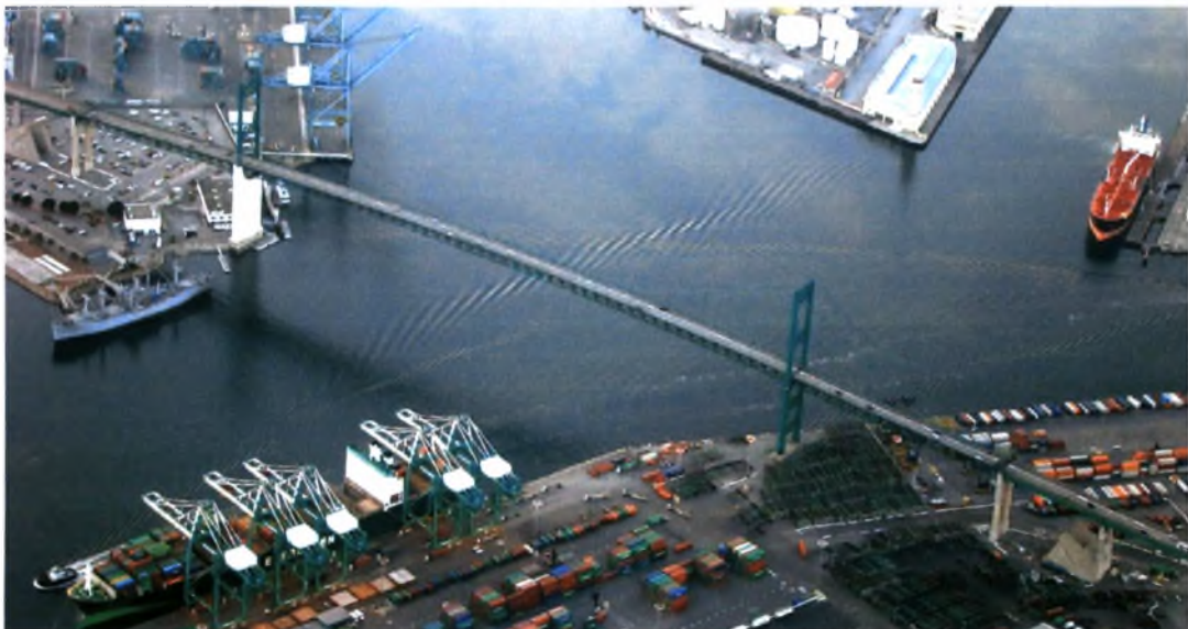
Figure 17: View of Vincent Thomas Bridge
