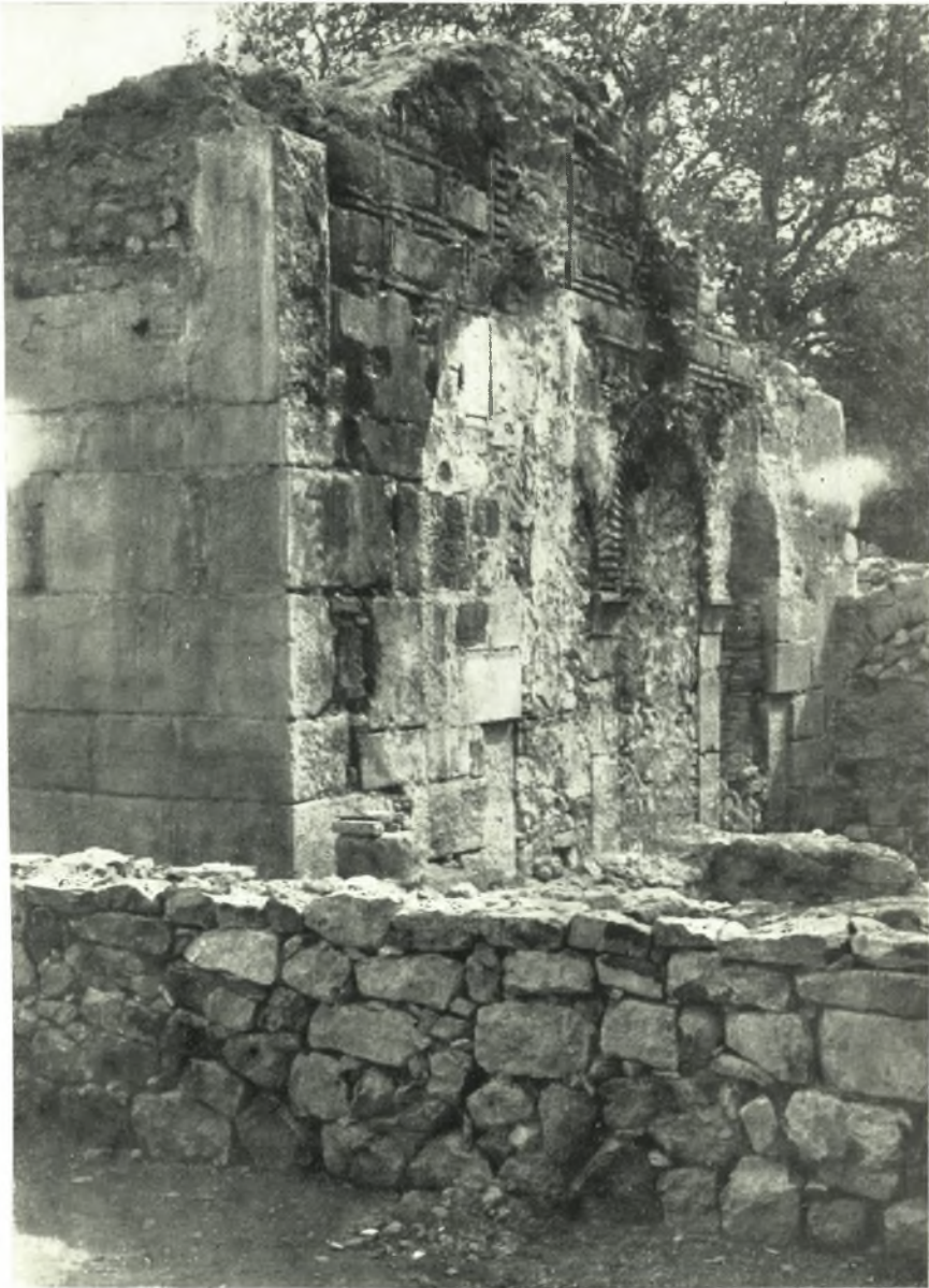
*Αποψις τῆς Τραπεζῆς ἀπὸ ΒΔ. πρὸ τῶν ἐργασιῶν ἀναστηλώσεως.
