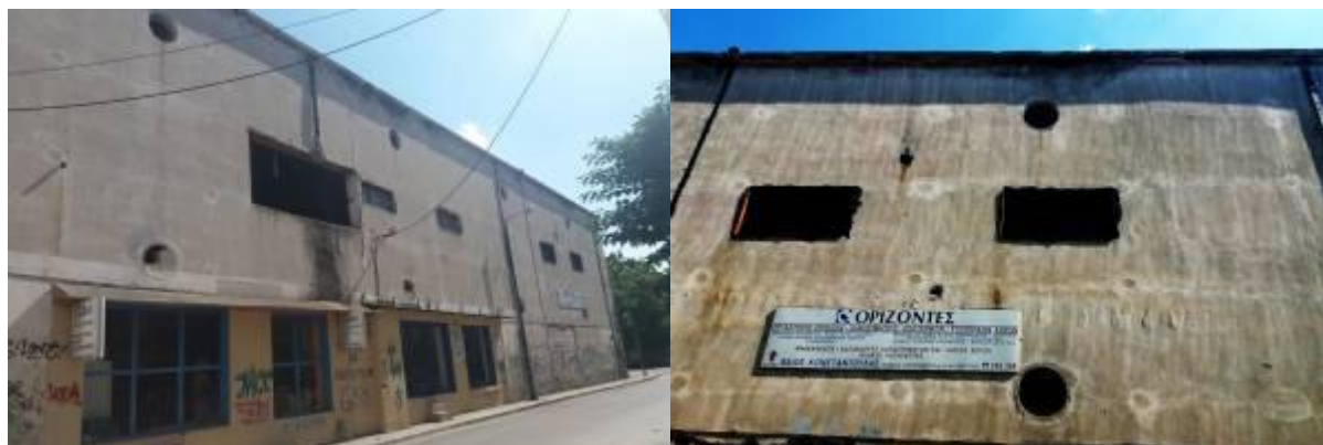
Figure 6.17 Infrastructure of Former Cold Storage Facility
