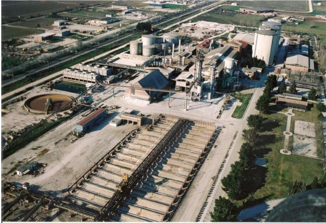
Figure 7.4 Overview of the Old Sugar Factory today
