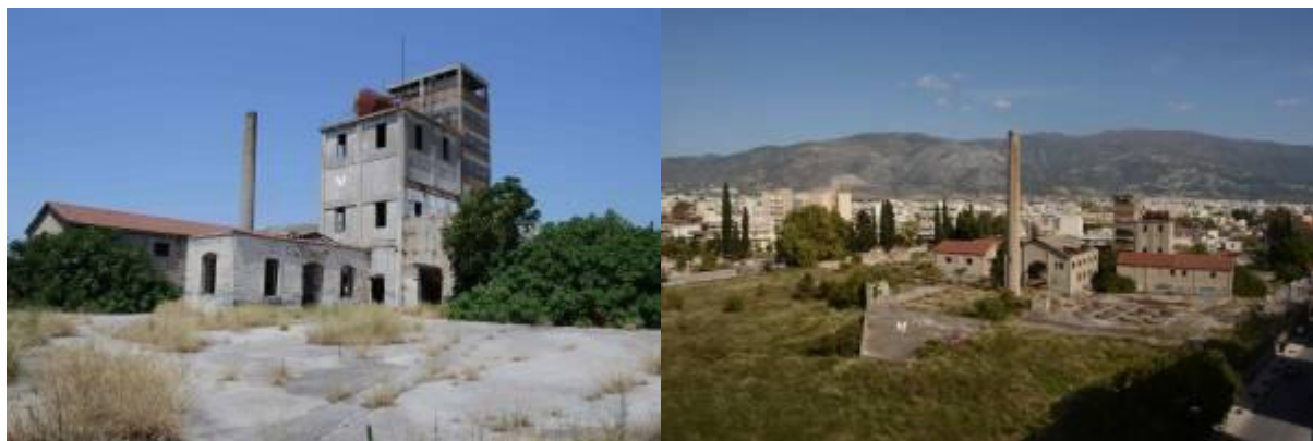
Figure 6.6 Infrastructure of Anagnostou Distillery Industrial Complex
