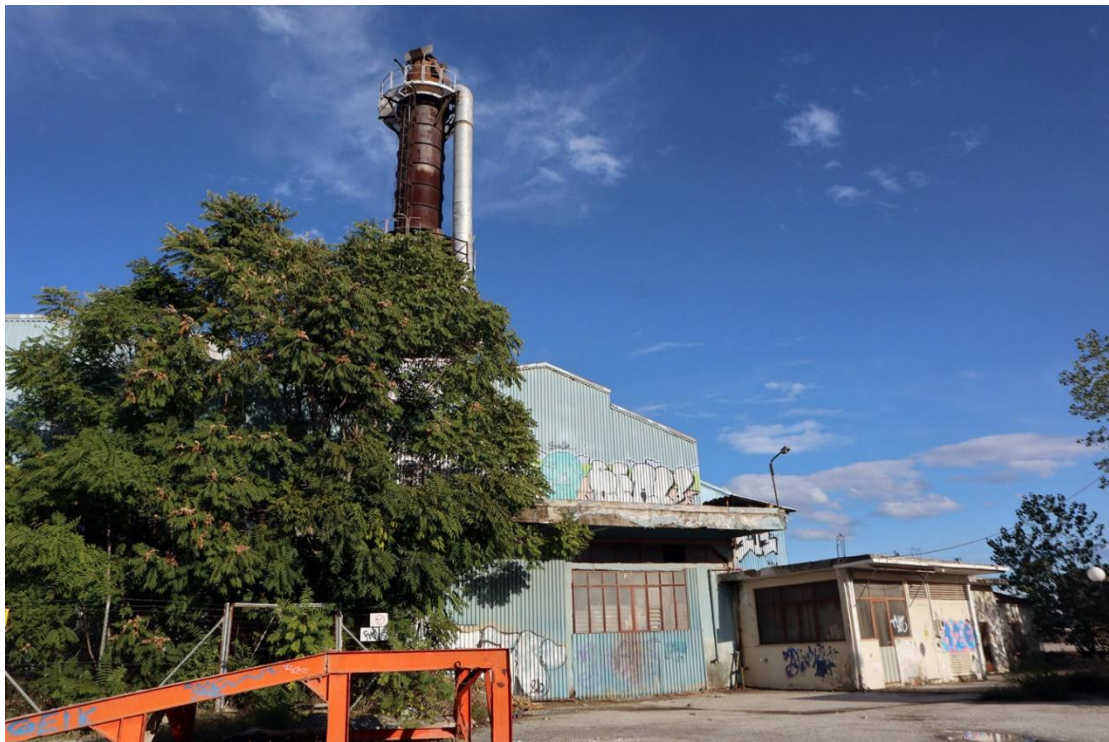
Figure 7.2 Current state of the Old Sugar Factory
