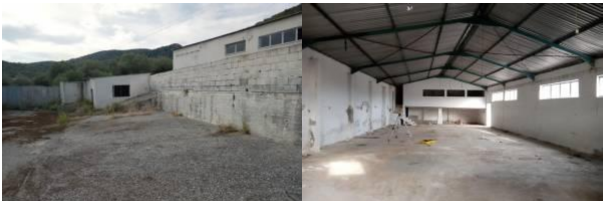
Figure 6.3 Infrastructure of Daferrera Fish Processing & Packaging Industry
