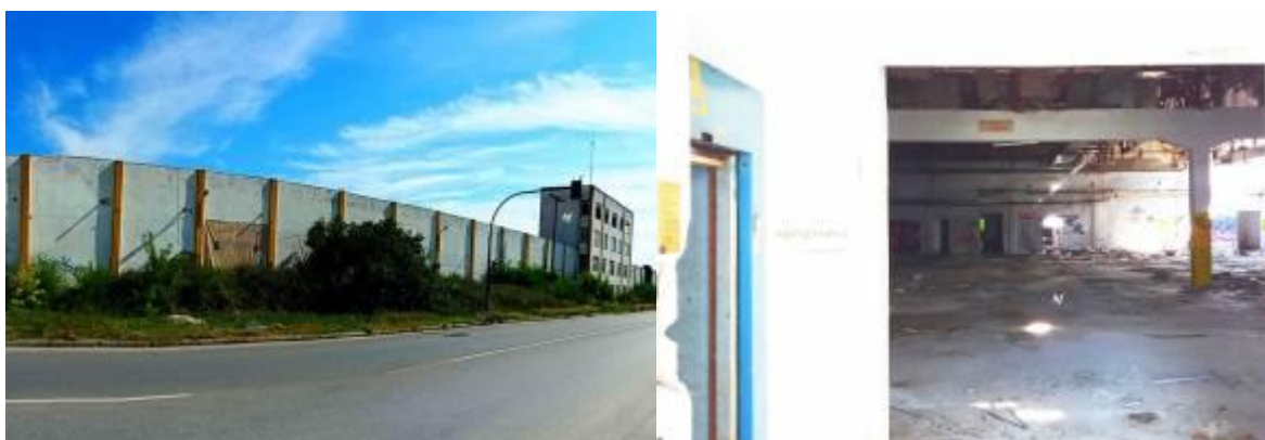
Figure 6.19 Infrastructure of Former Afoi Magrizou S.A. Textile Factory
