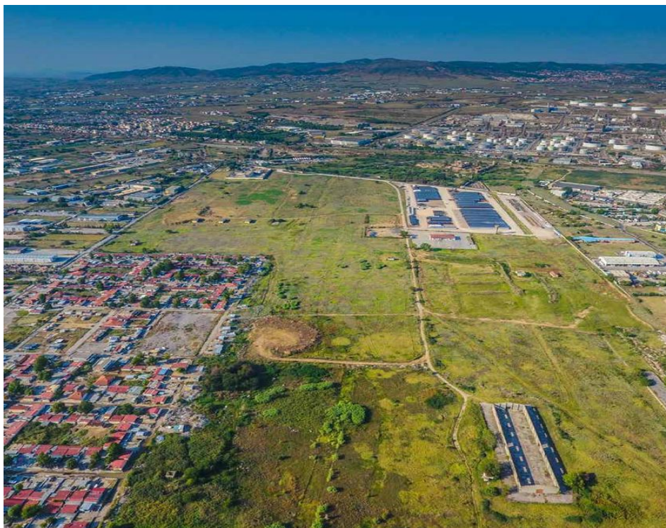
Figure 3.10 Overview of Gonos Logistics center
