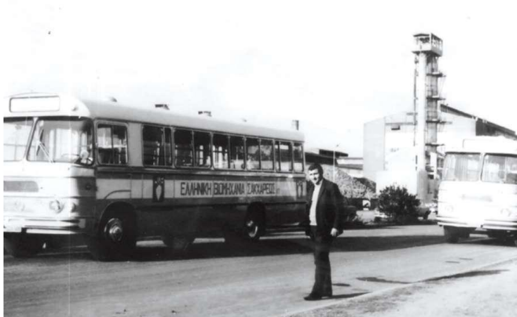
Figure 7.1 Historical photo of a worker outside the Old Sugar Factory
