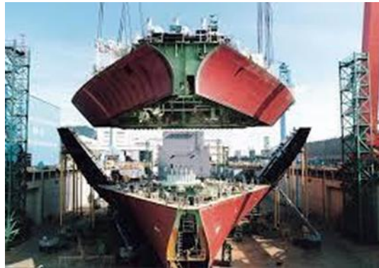
Figure 10: Prefabrication process in shipyard.
