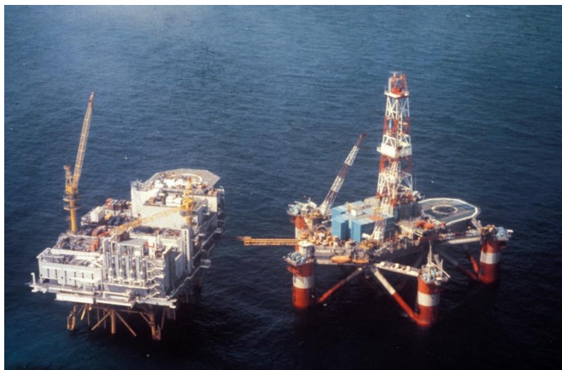
Figure 69: The Alexander L. Kielland offshore platform.
