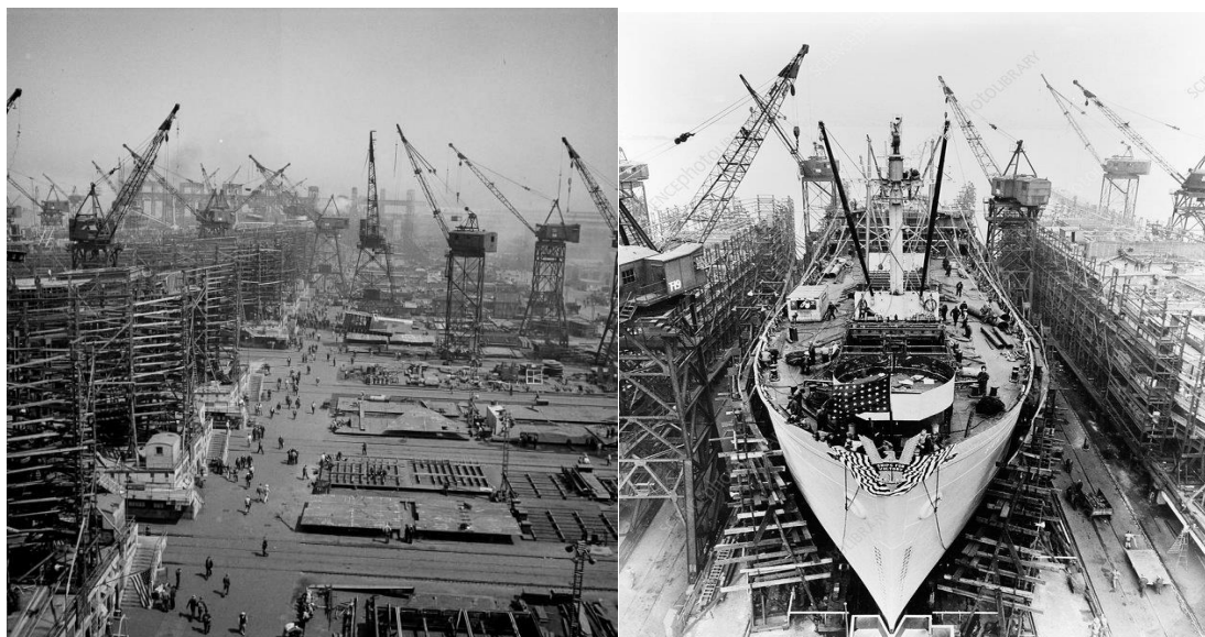
Figure 51: Liberty ships under construction.
