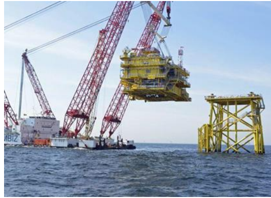
Figure 14: Installation of an offshore platform.
