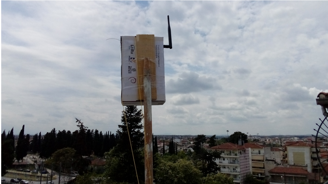
Figure 3.3: Position of the fixed base station on the sixth floor of an apartment building.
