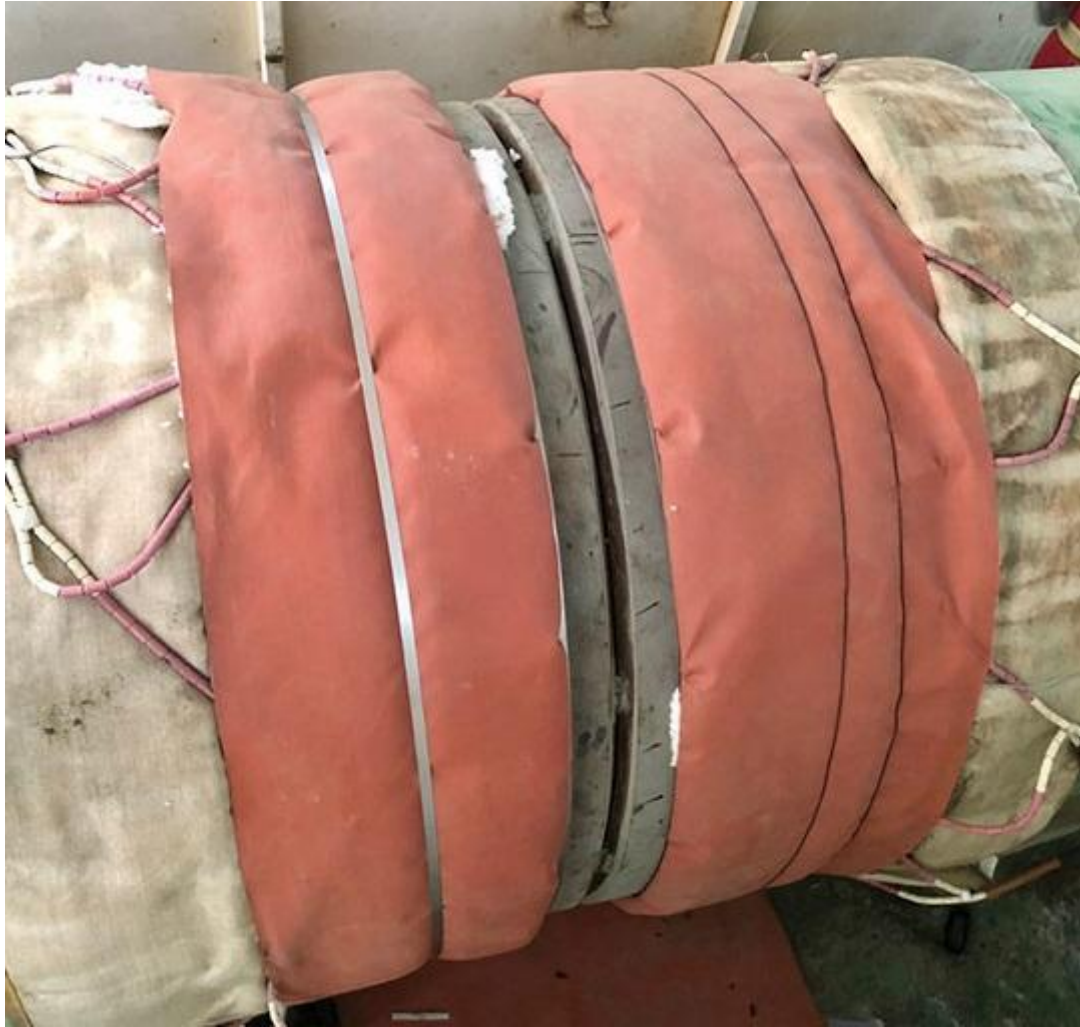
Figure 5.5 Preheating with electrical blankets [28]
