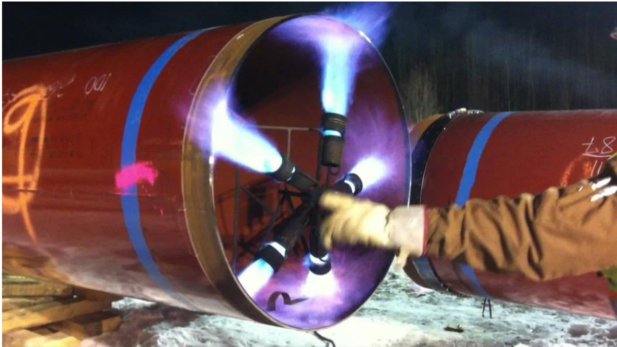
Figure 5.4 Preheating procedure with flame in pipe welding [27]
