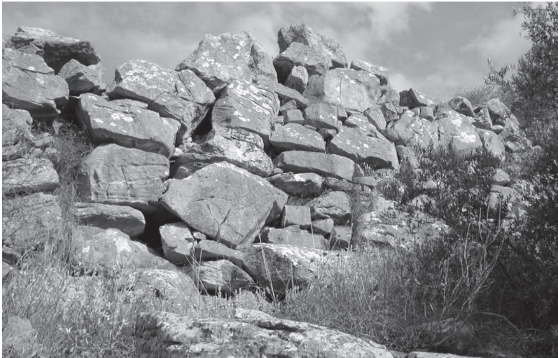
Fig. 3. The western wall near C. Elevation is over 3m high.
