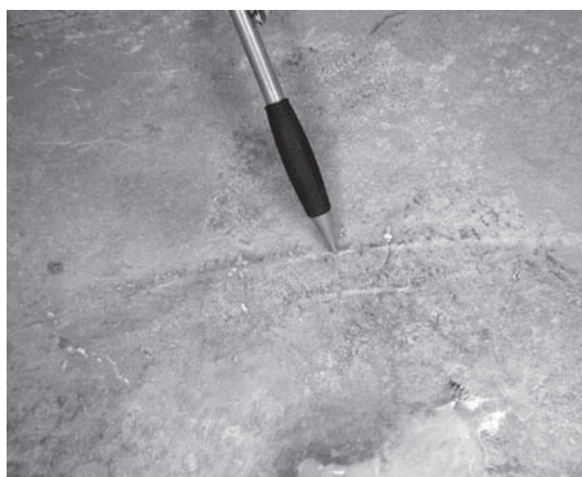
Fig. 4. Double line is obvious all around vessel A.
