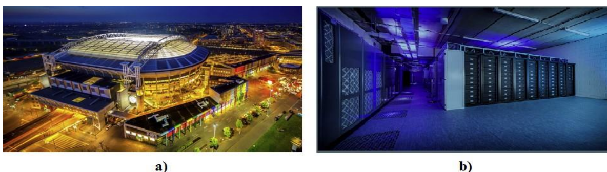
Figure 38: a) Amsterdam's "Johan Cruyff Arena" multipurpose stadium, b) Racks with part of the 2.8 MWh energy storage system at the "Johan Cruyff Arena" [34].
