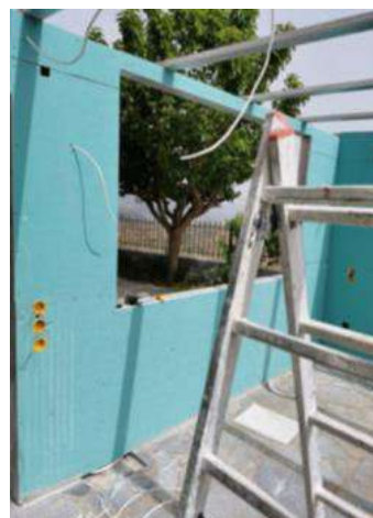
Picture 3: Electric installation works
