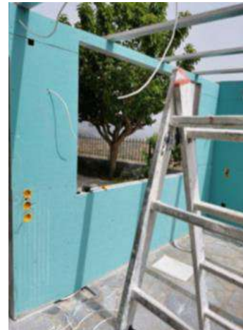
Picture 3: Electric installation works
