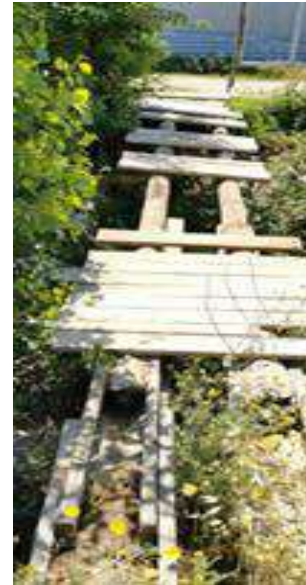
Picture 15: The constructed bridge
