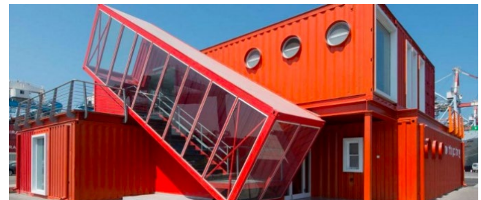
εικόνα 26: Angled shipping container houses a staircase for Israeli port office by Potash Architects
