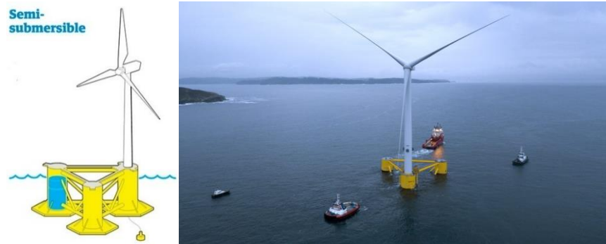
Figure 5: Main design concept of semi-submersible floating design wind energy platform (left), WindFloat Atlantic wind energy platform (right)
