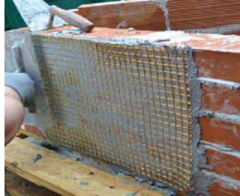
Σχήμα 2.7 Εφαρμογή των ΙΑΜ σε διάφορα δομικά μέλη ΟΣ και άοπλης τοιχοποιία. http://www.impresedilines.it/da-ruredil-le-soluzioni-antisismiche-certificate-aci549/ https://www.ildispariquotidiano.it/it/consolidamento-antisismico-oggi-giornata-di-studi-ruregold-a-ischia/ https://www.ingegneri.cc/consolidamento-statico-frcm-le-istruzioni.html https://www.researchgate.net/figure/Application-of-a-PBO-FRCM-strengthening-to-a-masonry-substrate_fig2_338279897
