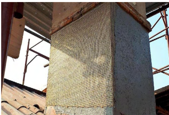
Σχήμα 2.7 Εφαρμογή των ΙΑΜ σε διάφορα δομικά μέλη ΟΣ και άοπλης τοιχοποιία. http://www.impresedilines.it/da-ruredil-le-soluzioni-antisismiche-certificate-aci549/ https://www.ildispariquotidiano.it/it/consolidamento-antisismico-oggi-giornata-di-studi-ruregold-a-ischia/ https://www.ingegneri.cc/consolidamento-statico-frcm-le-istruzioni.html https://www.researchgate.net/figure/Application-of-a-PBO-FRCM-strengthening-to-a-masonry-substrate_fig2_338279897
