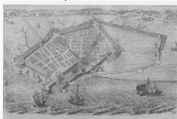
Expansion and Fortification
