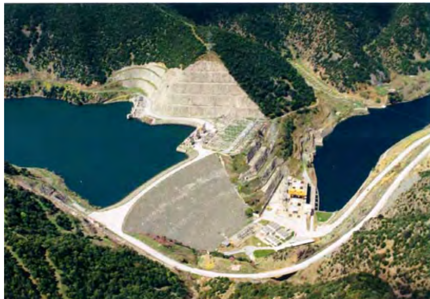
Figure 4.2: Sfikias pumped-storage plant
