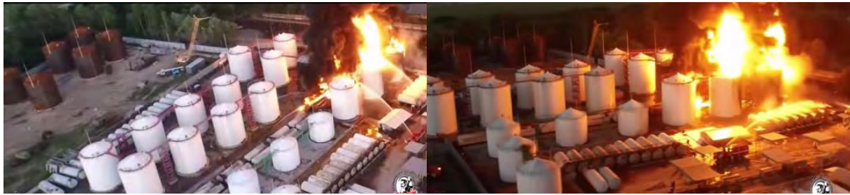
Figure 1-1 Kiev oil tank fire event.
