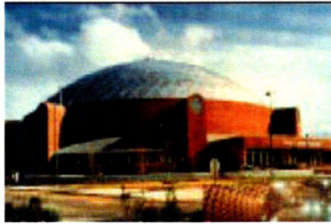
Fig. 1.4 The roof structures for arenas and gymnasiums are usually 6063 or 6061 extruded tube, covered with 5xxx alloy sheet. [2]
