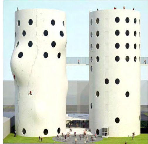
04 Abandoned Silos transformed into a climbing gym
