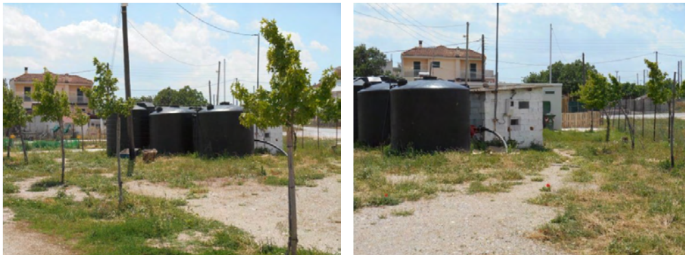
Image 10: The water reservoirs and the space of drilling
