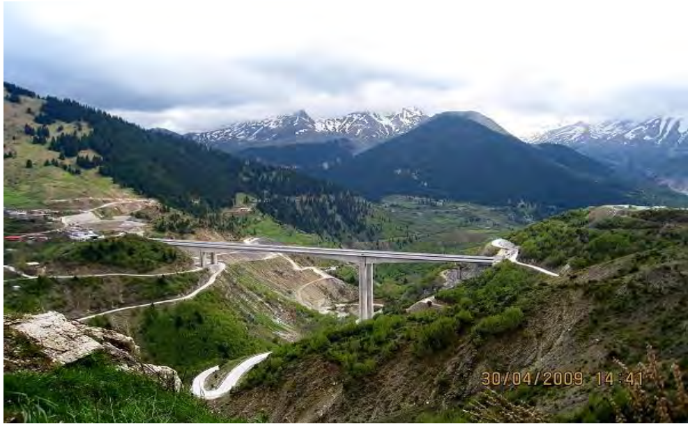
Figure 3.2: The ravine bridge of Metsovo
