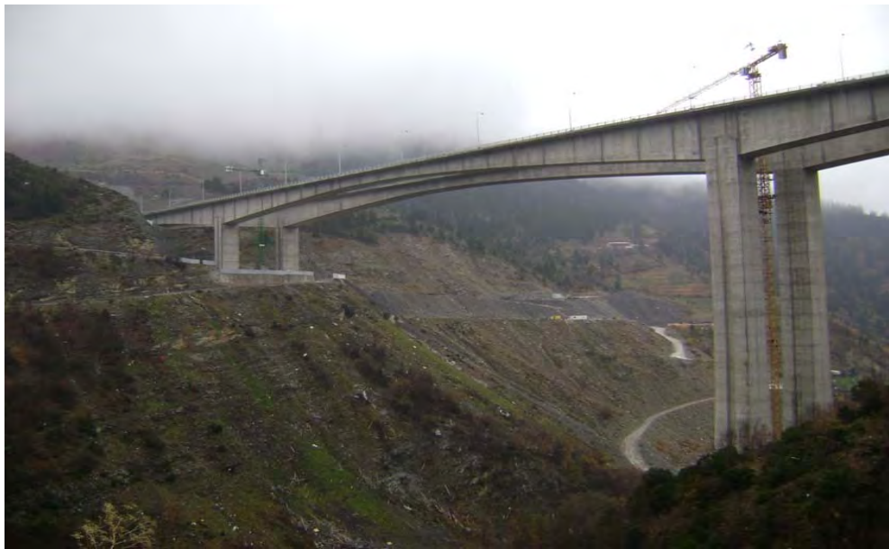
Figure 3.3: The ravine bridge of Metsovo
