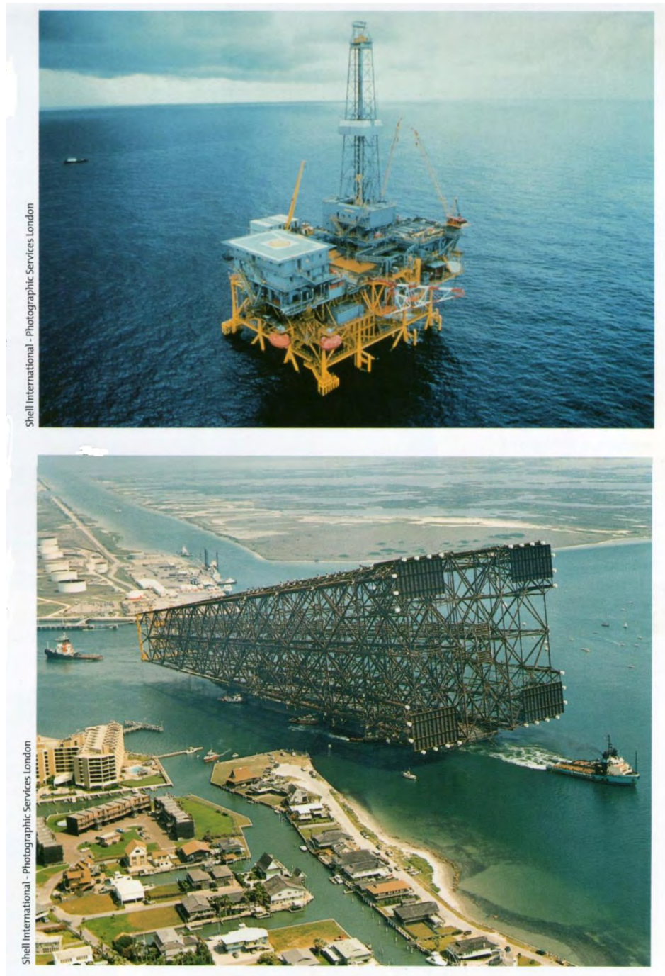
Figure 2 Bullwinkle platform decks in the Gulf of Mexico- Bullwinkle's substructure
