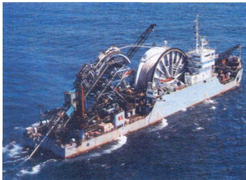
Figure 73: Pipe installation by reeling method.
