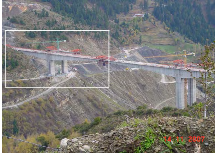
Figure 3.13: General view of the under construction Metsovo ravine bridge (November 2007)
