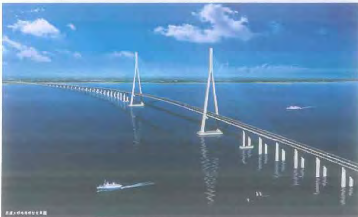
The Sutong Bridge (China)
