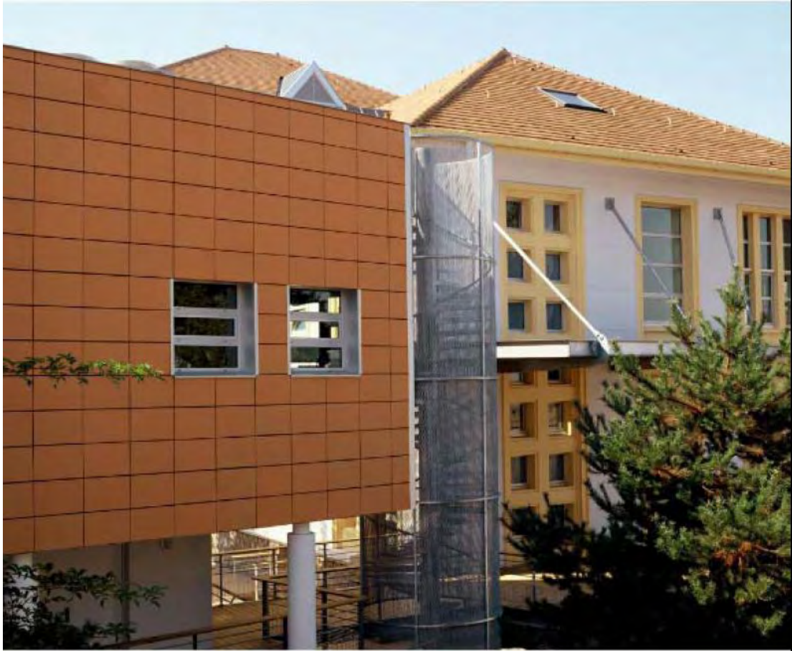
Figure 3-1 Photo of a two-story house with double façade of ceramic tiles (adapted from [135]).
