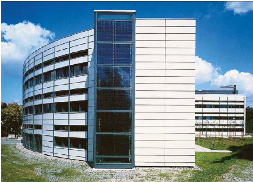
Figure 2-6 The PV façade at the office building of the Fraunhofer ISE, Freiburg. (adapted from [8])
