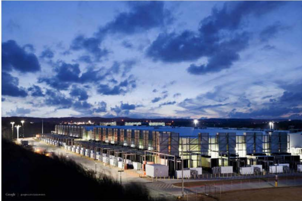
Figure 10: A Google data center outside Atlanta, Ga.
