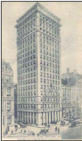
11. To American Surety Building.
