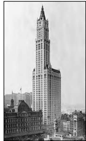
14. To Woolworth Building.
