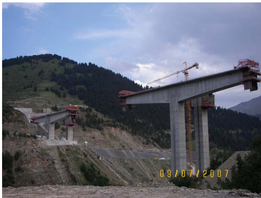
Figure 3.3: M3 Cantilever construction phase on 9/7/2007
