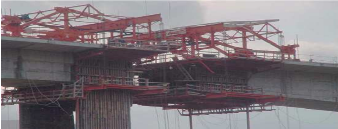
Figure 2.4: Key of central span of under construction Metsovo ravine bridge
