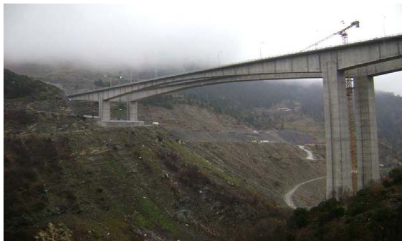
Figure 1.3: General view of Metsovo ravine bridge.
