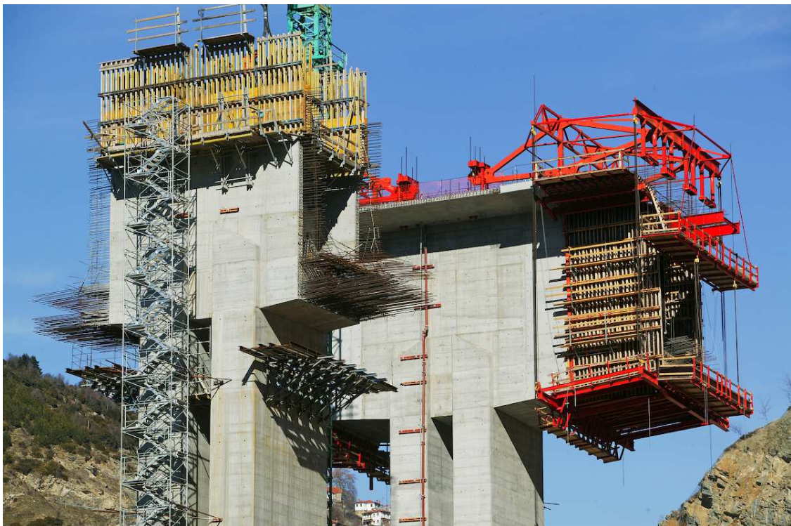
Figure 2.7: Longitudinal section of under construction Pier M3of Metsovo ravine bridge
