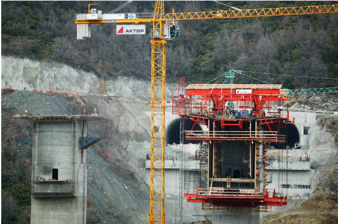
Figure 2.6: General view of under construction Pier M3of Metsovo ravine bridge
