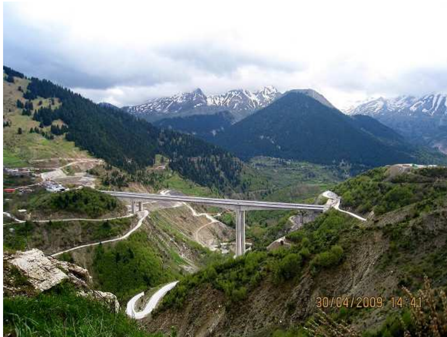
Figure 2.1: General view of Metsovo ravine bridge.
