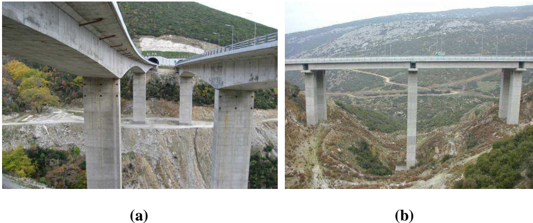
Figure 1.1: (a) Transverse Section of G2 Kavala Bridge , (a) Longitudinal Section of G2 Kavala Bridge.
