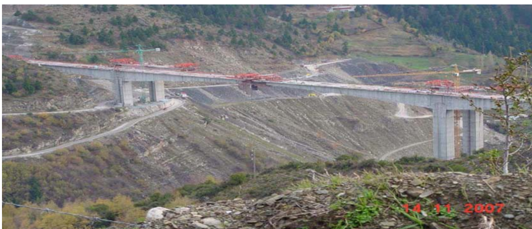
Figure 2.5: General view of under construction Metsovo ravine bridge (November 2007)
