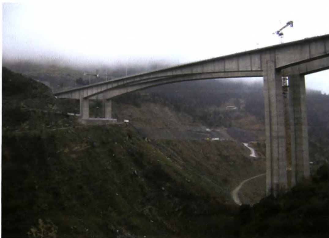
Figure 5.20: General view of Metsovo ravine bridge (November 2008)
