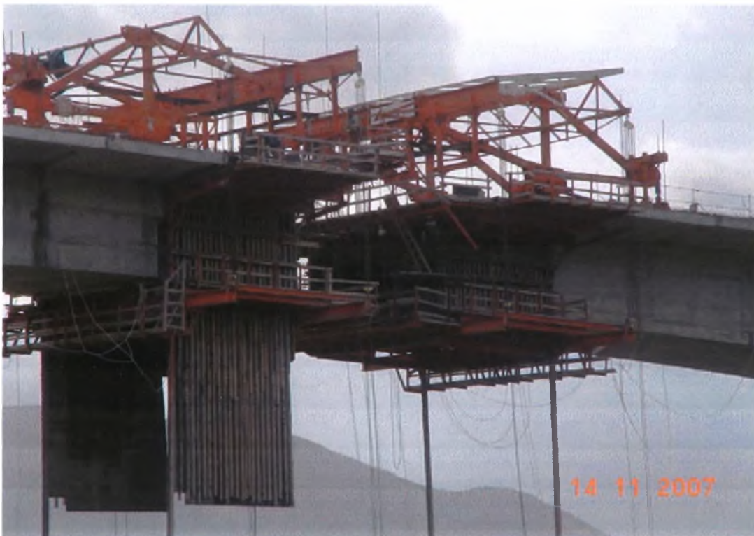
Figure 5.19: Key of central span of under construction Metsovo ravine bridge
