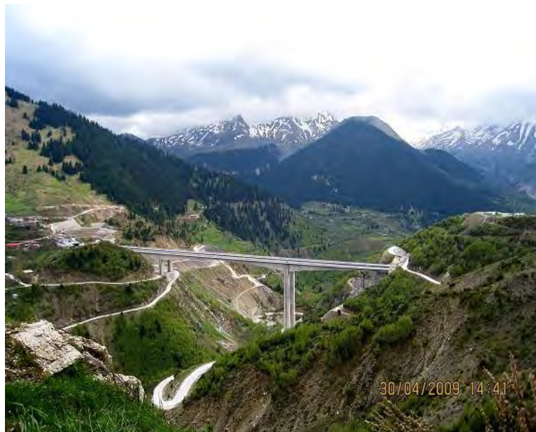
Figure 4.2: The ravine bridge of Metsovo
