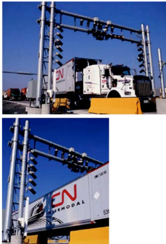
Figure 27. Automated Gate Systems at CN intermodal facility in Brampton, from CN International.
