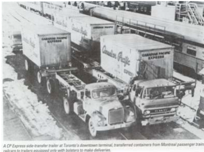
Figure 1. First container transports
