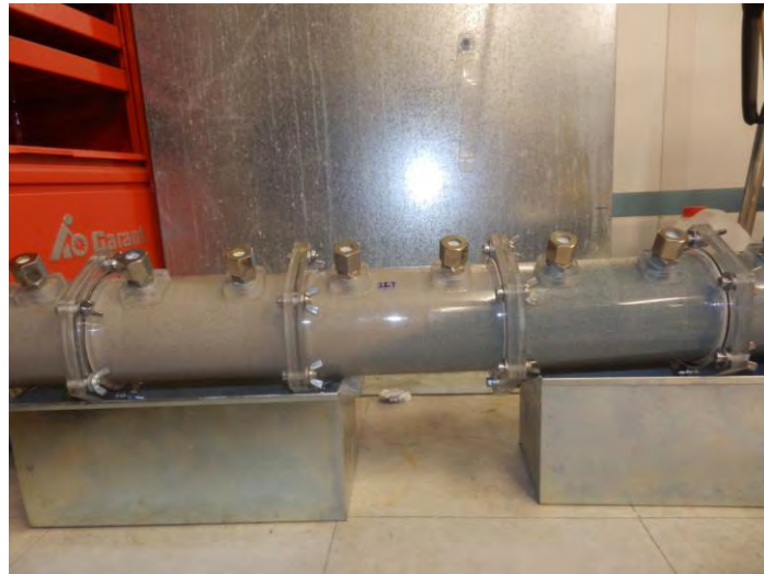
Figure 5.53 View of CS front location during the horizontal injection test.
