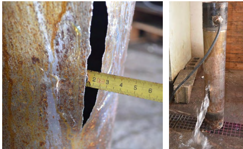
Figure 3-62: Rupture of perfect \text{Ø}165/3 pipe specimens; (a) thickness wall reduction at the critical region and (b) the location of the rupture.
