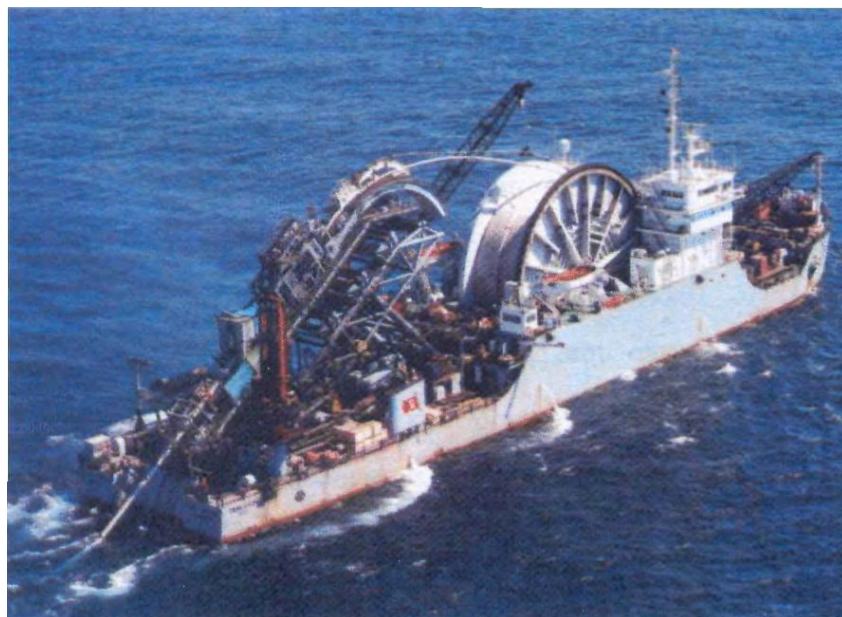
Figure 73: Pipe installation by reeling method.
