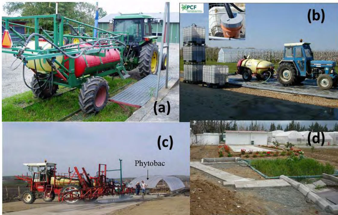
Figure 1.18. Photos of the main types of biobed systems used in Europe: (a) original driver over biobed system; (b) biofilter system used in Belgium; (c) Offset type Phytobac system originated from France, and (d) UK offset type biobed system in Cyprus.
