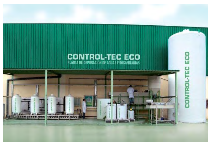
Figure 1.19. The CONTROL-TEC ECO® system used for the treatment of wastewaters from the fruit packaging industry.
