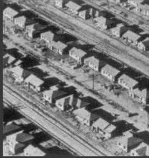
Subdivision under construction, near Los Angeles. Photos William Garnett
