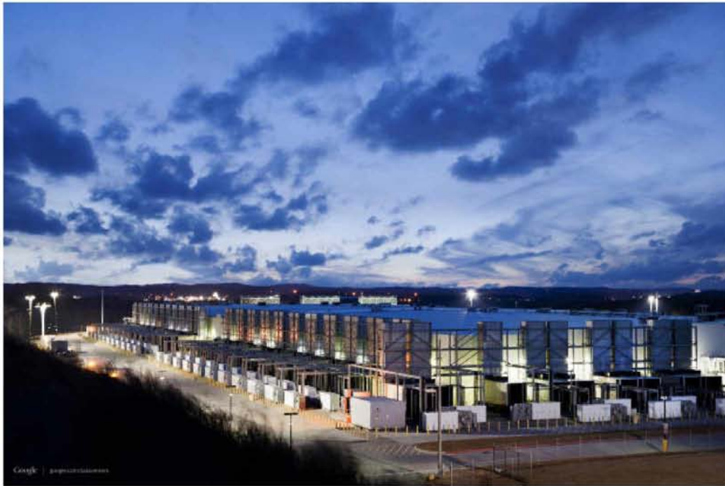
Figure 10: A Google data center outside Atlanta, Ga.
