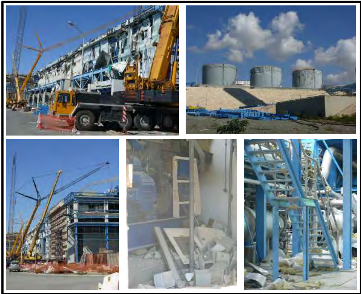
Figure 1. Pictures from Vasilikos Power Station (October 13th, 2011).
