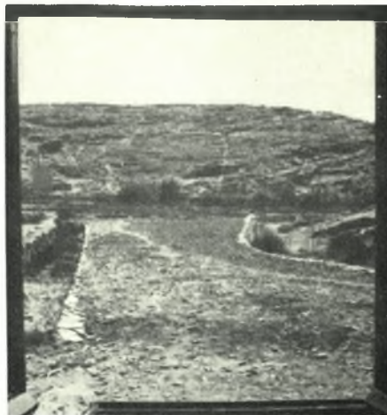
Kea. Ayia Irini : a. Rooms XIII and XV. Repairs and buttresses, marked with whitewash, b. Guardhouse and workrooms, from the South, c. View from east window of guardhouse towards the new road built by the excavators in 1963 - 1964. This is the public road from Vourkari and Korissia
