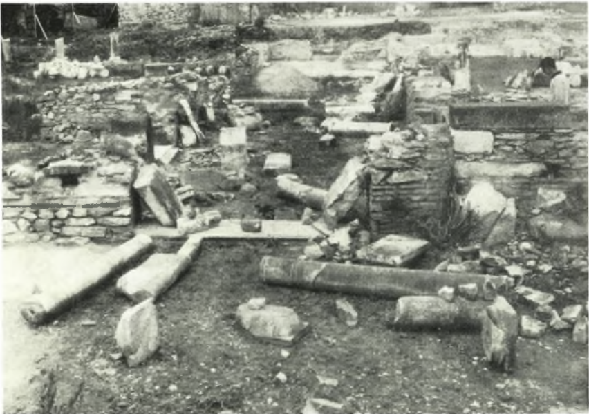
β. Ὁ ἐξωνάρθηξ πρὸ τῶν ἐργασιῶν (ἀπὸ Νότου).
